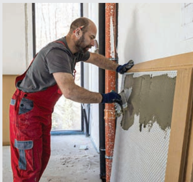
GLUING THE SLAB
