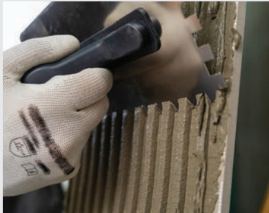
GLUING THE SLAB
