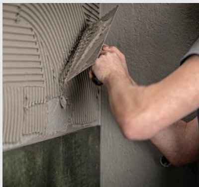
GLUING THE SUPPORT
