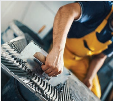
GLUING THE SLAB
